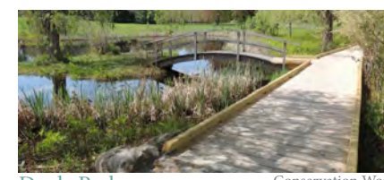
Doyle Park Conservation Works
